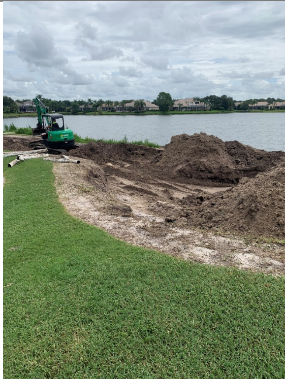
Bunker Backfill Stockpile
