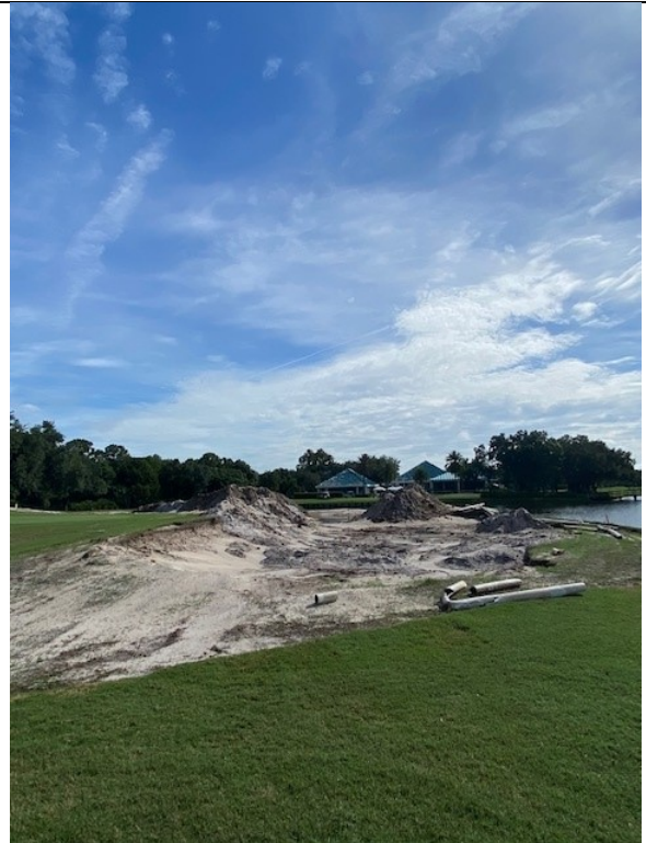
Bunker Excavation, Old Drainage Removal and Sand Stockpiling
