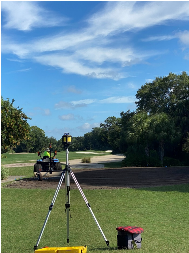
Laser grading
