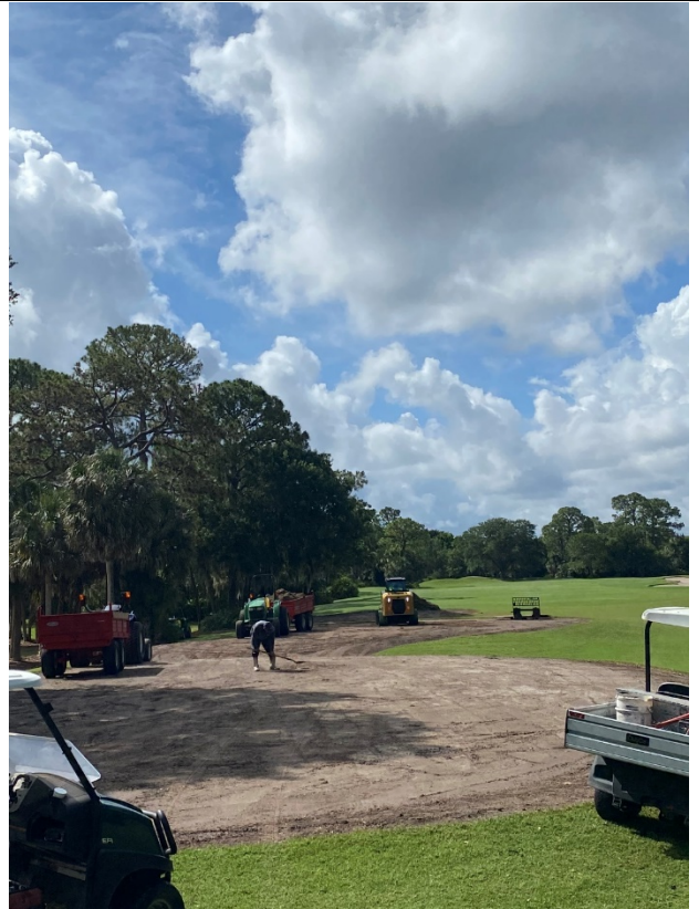
Hand grading preparing for sod
