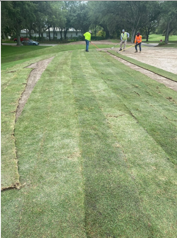
"Good" sod installation
